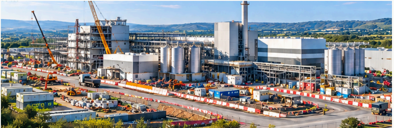
Shotton Mill, Deeside, a major £1.4 billion redevelopment for Eren.
